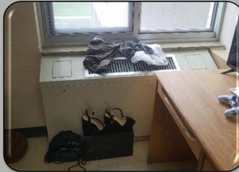
**Do not block your A/C unit with clothes, objects, furniture. It is critical that items remain at least 6 inches away from the HVAC unit to ensure proper ventilation.**
